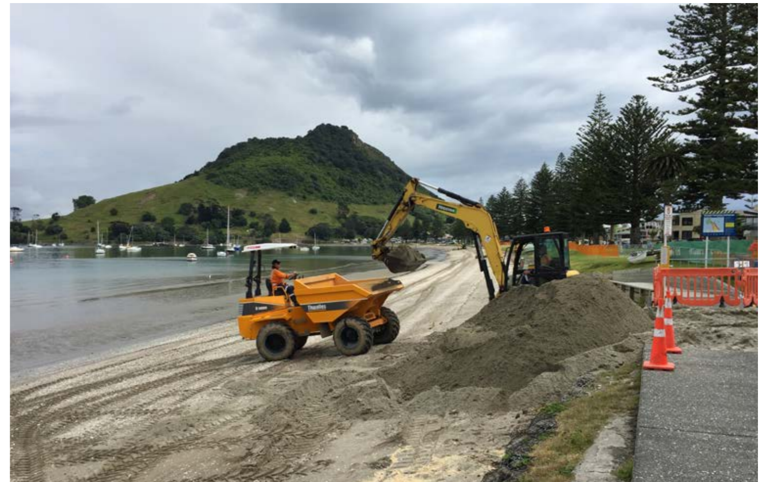
Sand replenishment at Pilot Bay beach, Mount Maunganui
