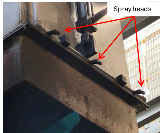
Dust suppression sprays on the coal silo discharge chute.
