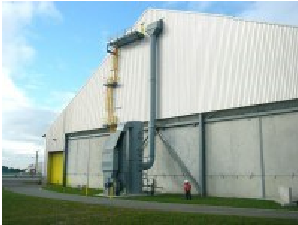
Figure 5.8: Centrifugal wet scrubber on Warehouse A (Image sourced from https://www.luehrfilter.com.au/Products/Wet-Scrubbers ).
