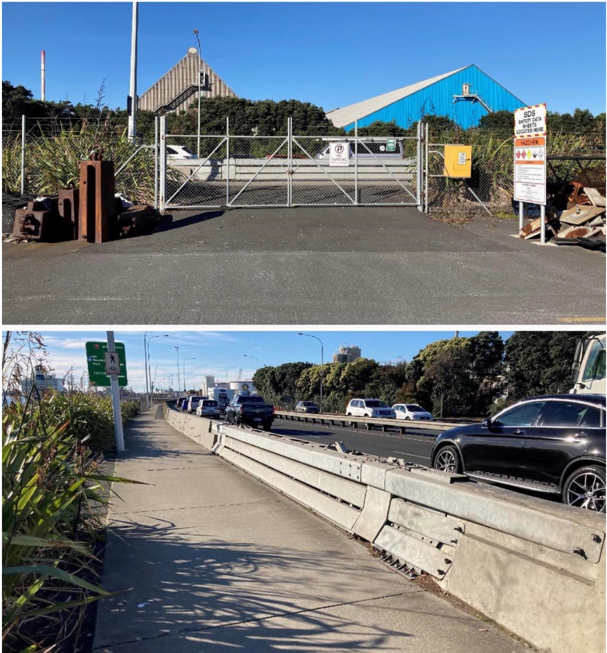
Figure 1: Emergency Access gates to Berth 16
