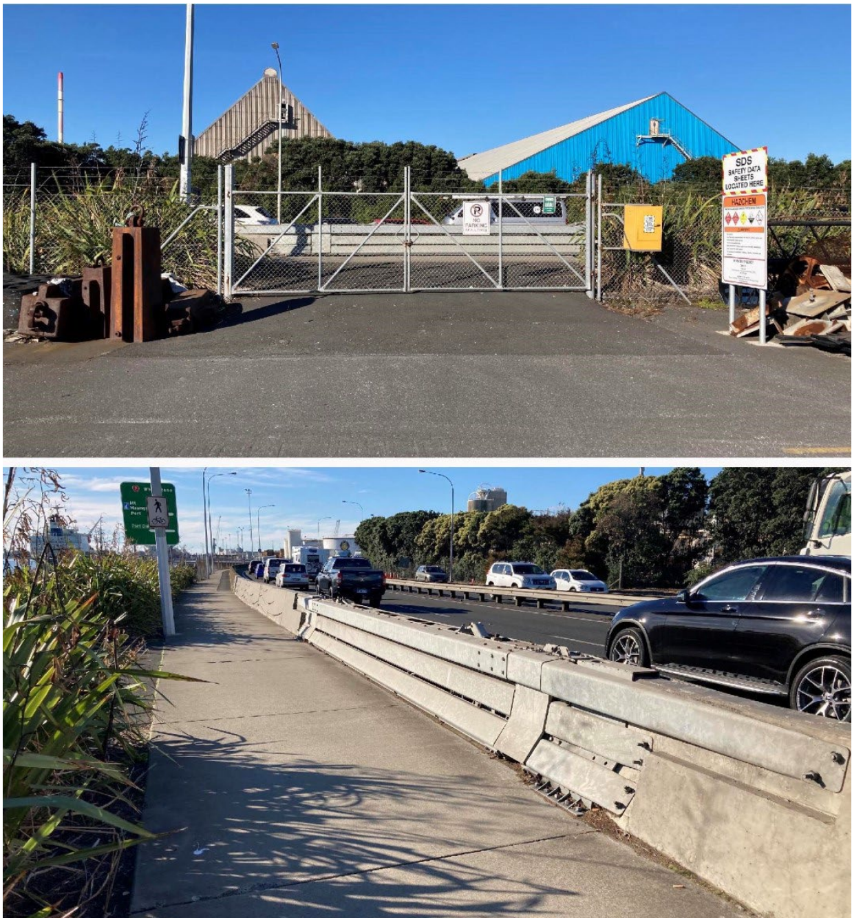
Figure 1: Emergency Access gates to Berth 16
