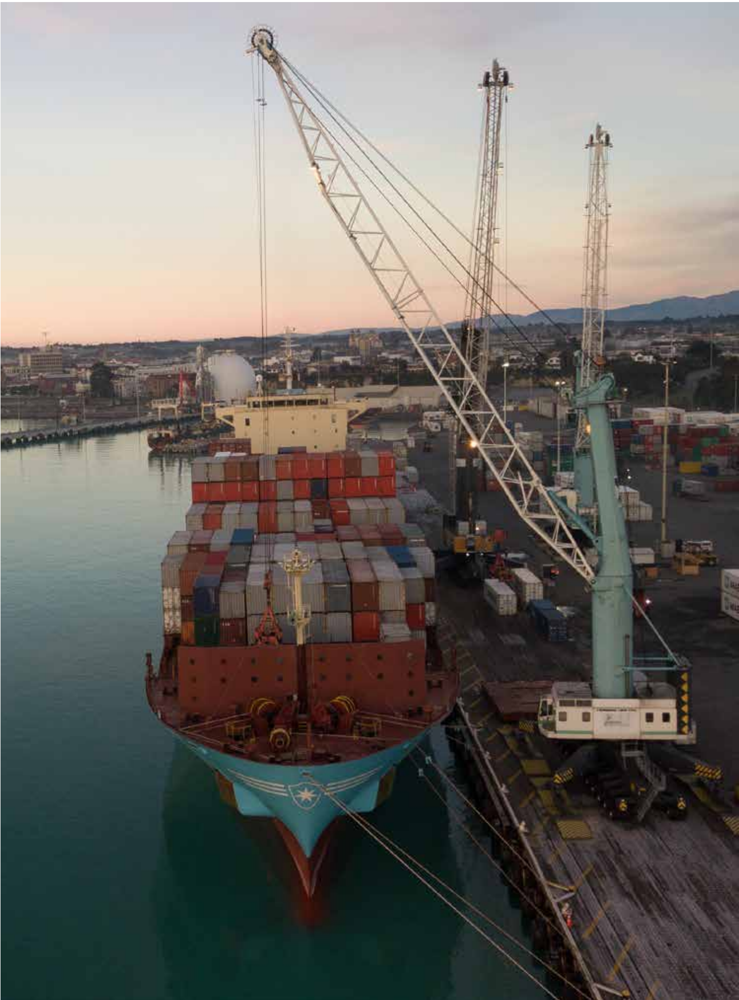
Timaru Container Terminal
